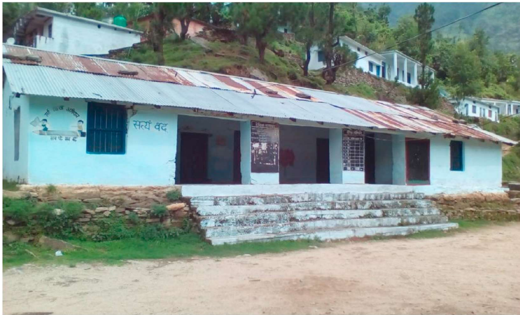
Fig. 5. Single storeyed Government Inter College building with CGI sheet as roofing material at Rau Lekh in Rudrapur district is built using stone foundation.
