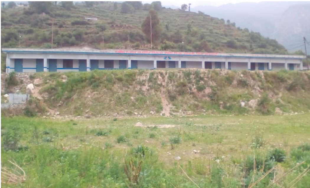
Fig. 7. Single storeyed Government Higher Secondary School at Raithal in Uttarkashi district having RCC slab as roof and built over sloping ground.
