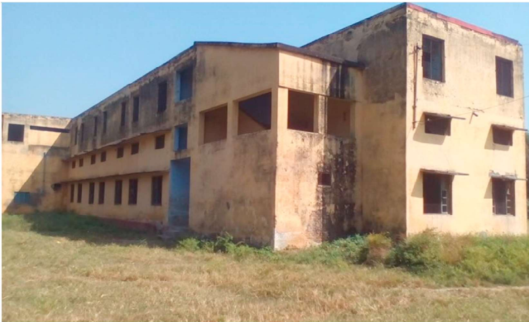
Fig. 11. Asymmetric building of Inter College at Jawalapur in Haridwar district.
