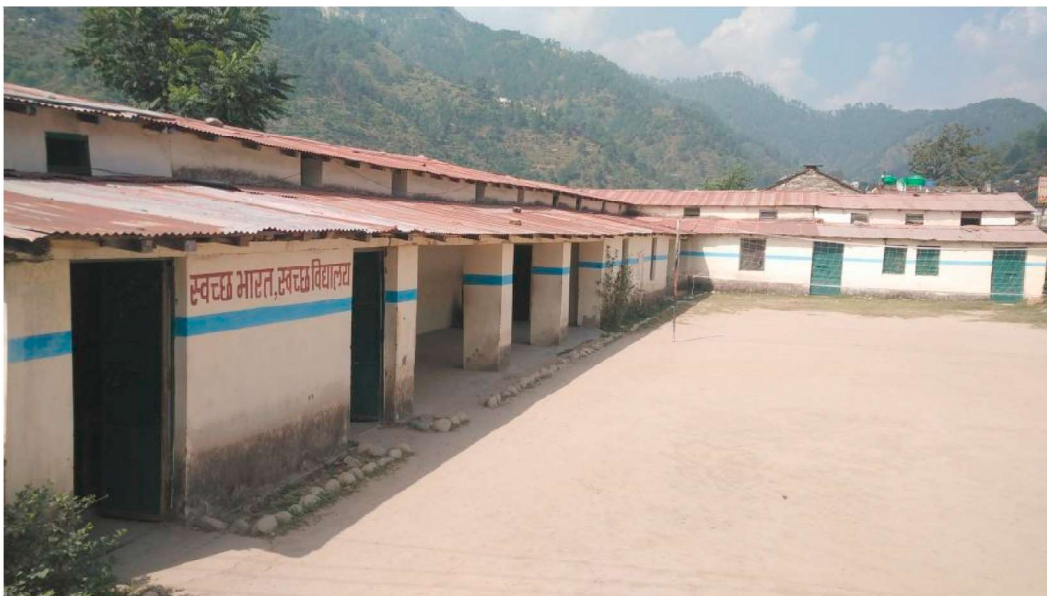
Fig. 3. Single storeyed irregular masonry building of Government Inter College at Syunsi in Pauri Garhwal district having CGI roof.
