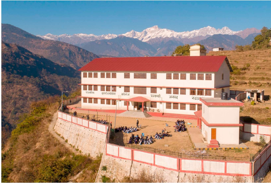
Fig. 4. Recently constructed three storeyed RCC Government Inter Collage building at Parkandi in Rudraprayag district having CGI sheets as the roofing material.
